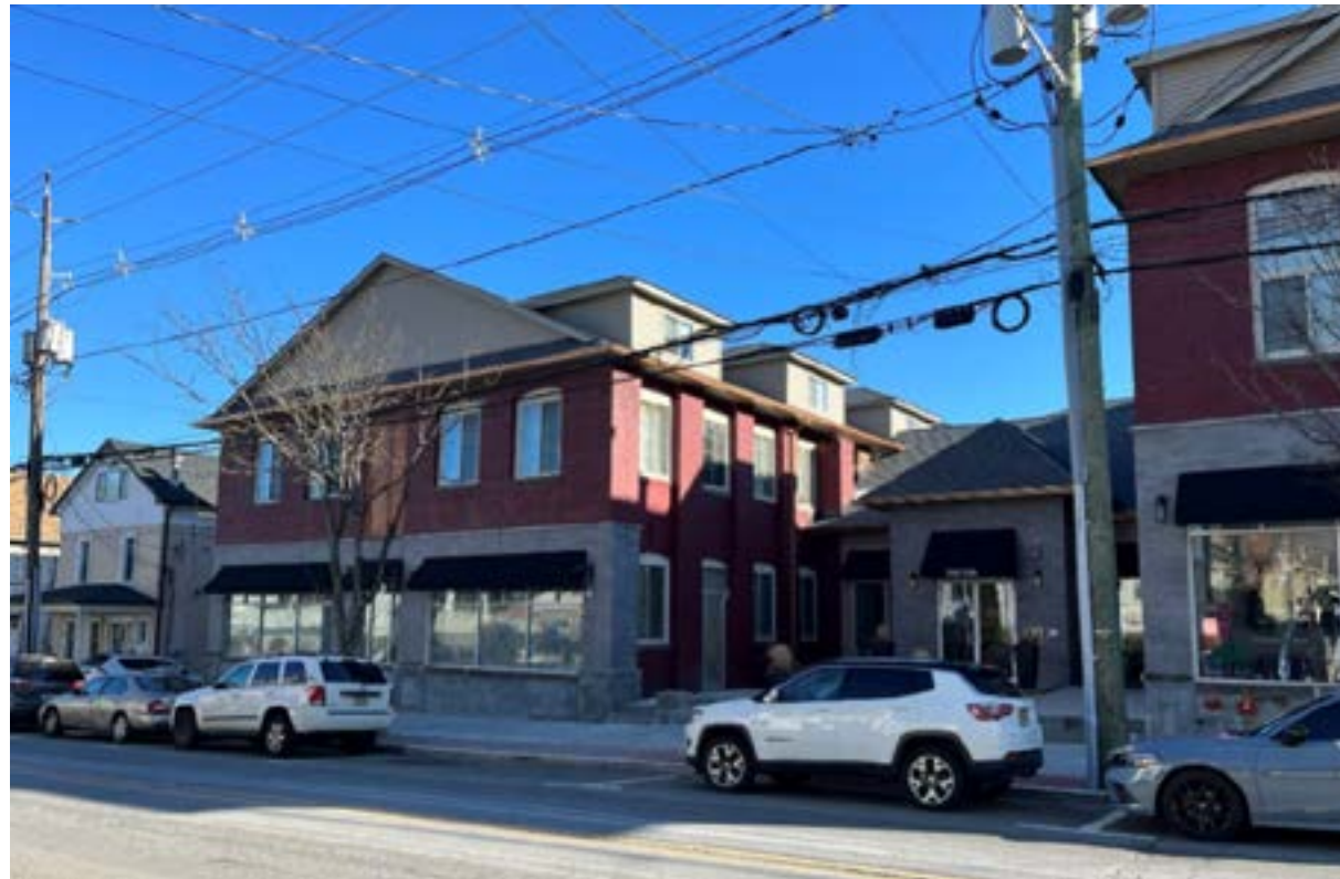
FIGURE 5. TWO ADJACENT LOTS IN PROSPECT PARK WERE DESIGNATED AS PROPERTIES IN NEED OF REHABILITATION; NOW THEY ARE HOME TO HOUSING AND RETAIL
