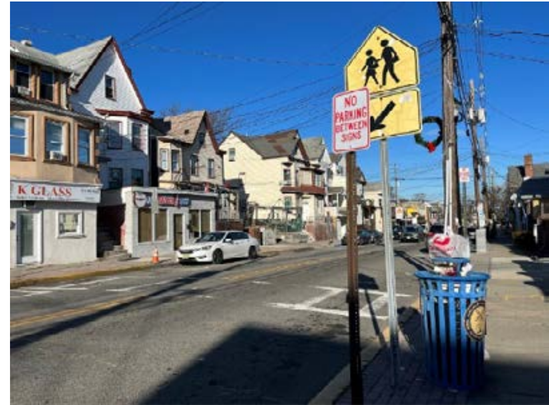
FIGURE 11 VIEW OF THE MARKED MIDBLOCK CROSSWALK FROM THE SOUTHERN EDGE OF NORTH 8 TH STREET. NOTE THE ON-STREET PARKING ON THE OPPOSITE SIDE AND THE OBSTRUCTED PEDESTRIAN SIGN IN FRONT OF THE BLUE TRASH CAN.
