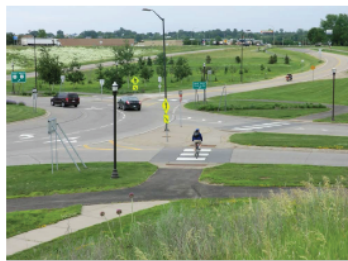
Example of a multi-lane roundabout.
