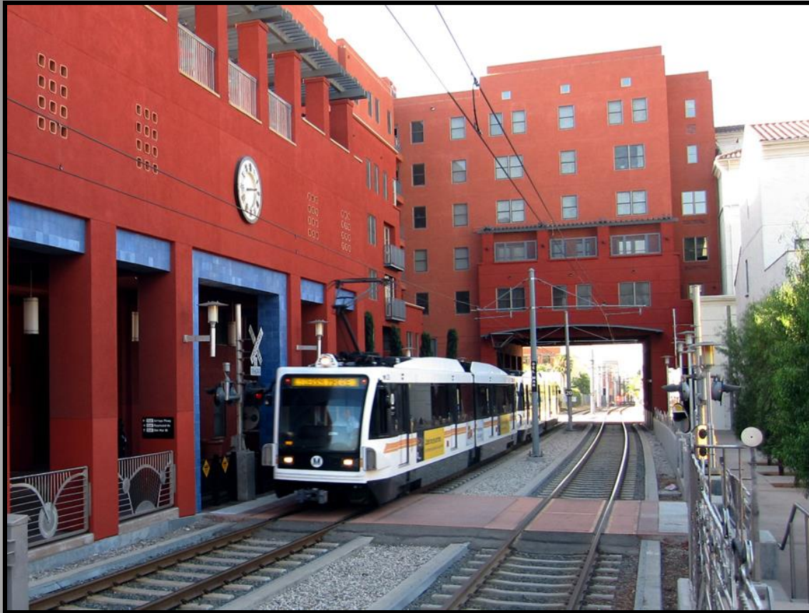
Del Mar Station, Gold Line LRT, Pasadena, CA
