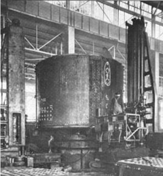
the Federal Shipbuilding Company's boiler shops showing special tools designed for the shells of Scotch boilers
