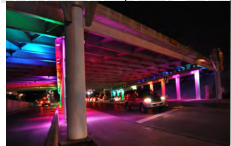
Route I-280 Underpass
