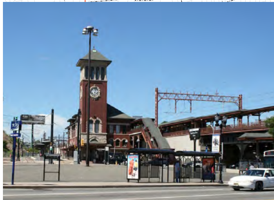
Newark Broad Street Station
