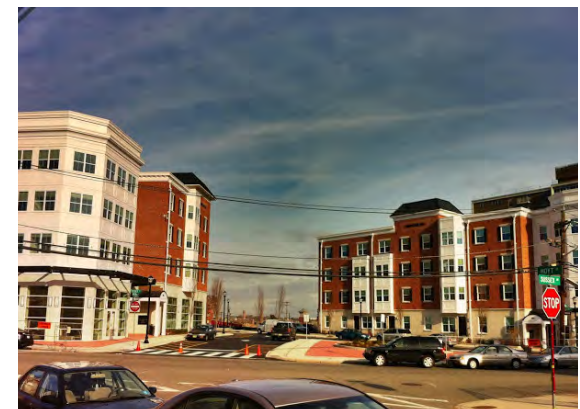
The rebuilding of Baxter Park after the demolition of Baxter Terrace
