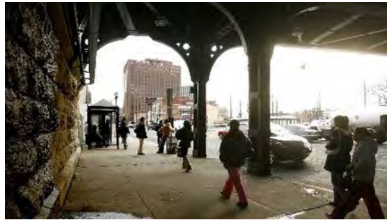
Under the existing overpass of I-280
