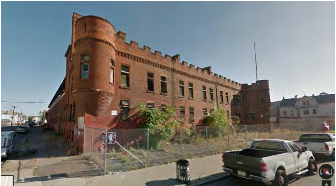
Figure 77. Paterson Armory Building
