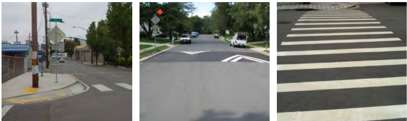
Figure 21. Traffic Calming Examples - (Left to right) Curb extensions, Speed Humps, High Visibility Crosswalks
