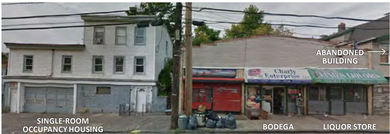
Figure 22. Incompatible Land-Use - This combination of adjacent land-uses may be a cause for increased crime in this location identified as hotspot "A" on Figure 13.
