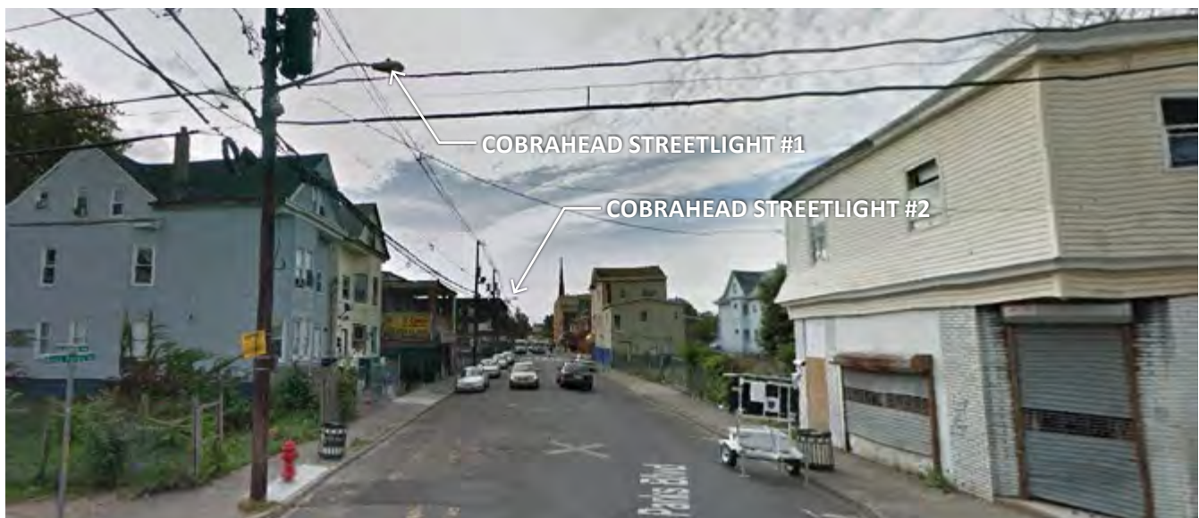
Figure 46. Typical street lighting shown between Godwin and Hamilton Avenue. Note that lighting is provided only at the intersection without any lighting provided throughout the middle of the block.
