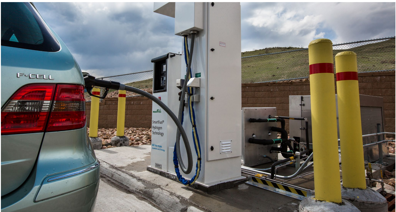
Photo by John De La Rosa, NREL 34236
